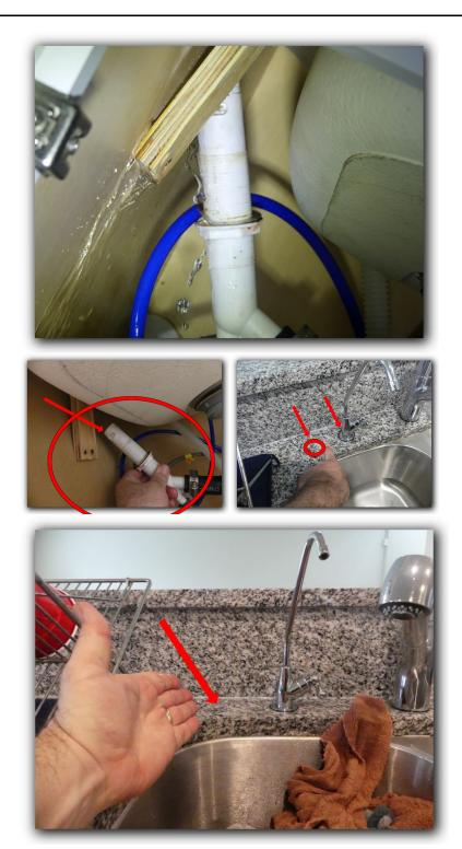
☑Sink leaks into cabinet below\*\*(Deficiency)\*\*
