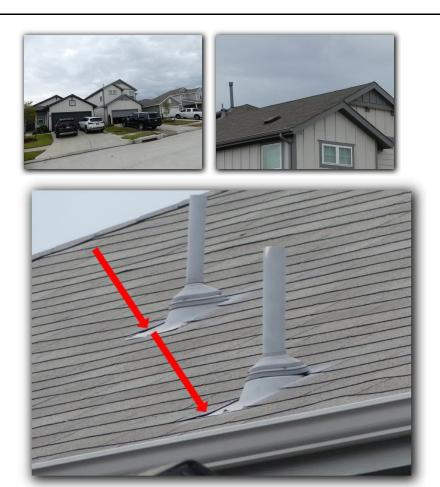
THERE IS SOME RAISED SHINGLES DUE TO PROTRUDING NAILS THAT NEEDS TO BE REPAIRED BY A ROOFING EXPERT.\*\*(Deficiency)\*\*
