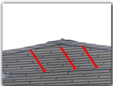
☑ Flashing is lifting, ill configured,\*\*(Deficiency)\*\*(Step flashing at the roof and wall intersections raised up that needs repairs by a roofing expert)\*\*(Deficiency)\*\*
