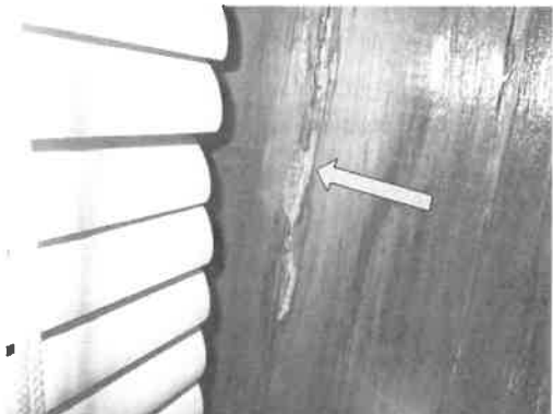
Water was standing on the sill of the left window on the front wall of bedroom 2, indicating water penetration between the window frame and the wall opening and/or dripping of excessive condensation.
