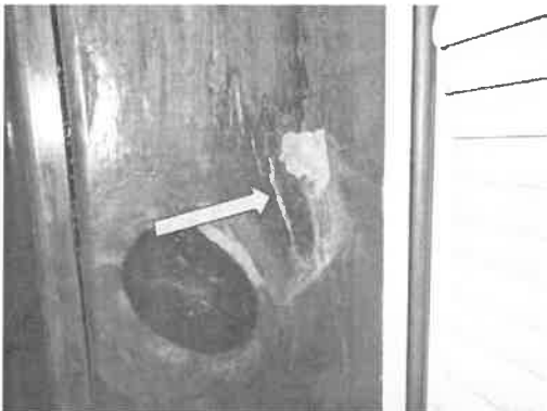
Water was standing on the sill of the left window on the front wall of bedroom 2, indicating water penetration between the window frame and the wall opening and/or dripping of excessive condensation.
