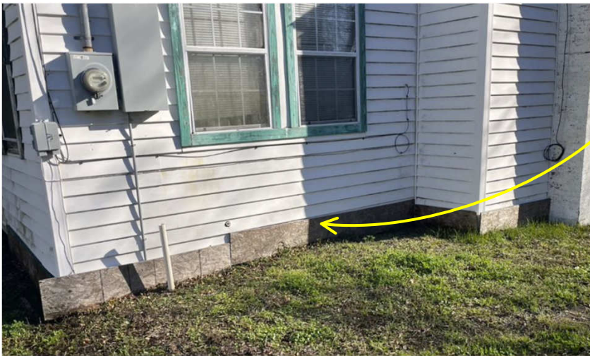
Standing water under east half of structure
