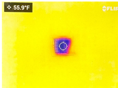
Cooling temperature reading at supply
