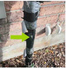
• "No sediment traps and/or drip legs noted on the natural gas lines at the mechanical equipment. Due to a change in construction standards, recommend plumber evaluate and repair as needed to meet todays standards."
