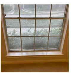
• Some window sills show evidence of moisture stains from condensation. Seal and monitor. (Dinning Room)
