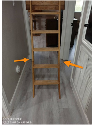
Improper slope
