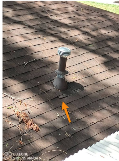
Lifted flashing
