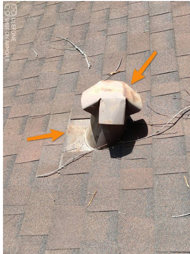
Corroded flashing
