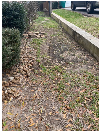
Example Right Exterior Wall
