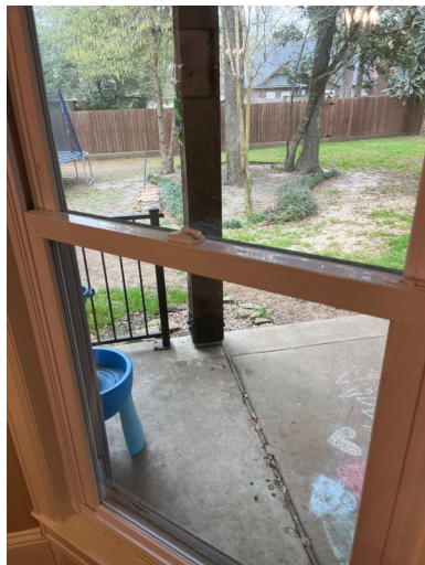
Example Rear Exterior Wall
