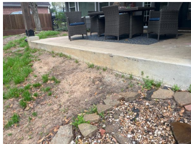
Example Rear Exterior Wall
