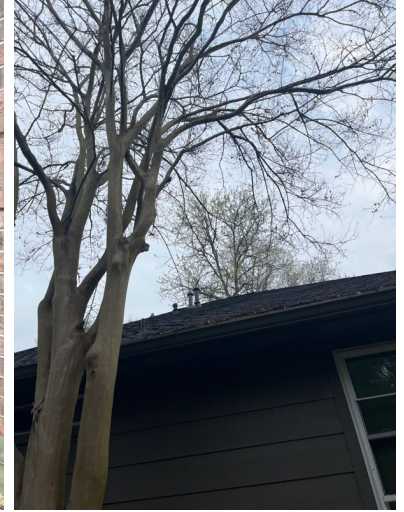
Example Rear Exterior Wall
