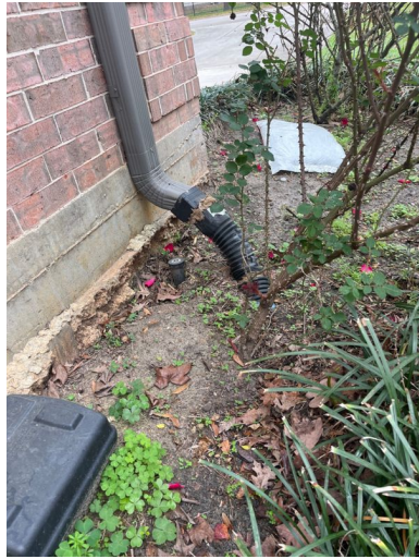
Example Left Exterior Wall
