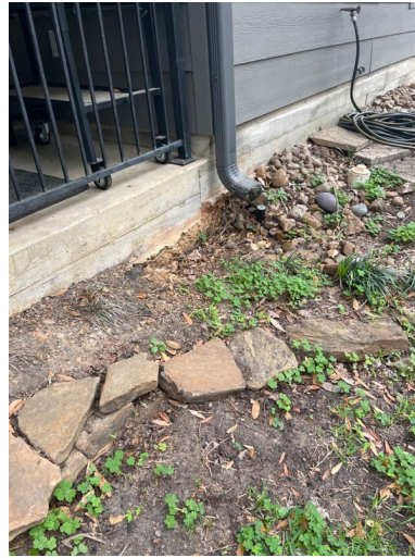
Example Rear Exterior Wall
