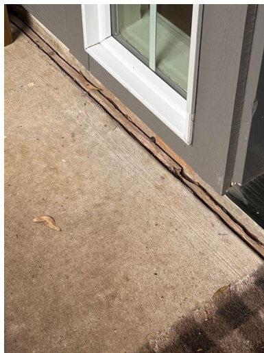
Example Rear Exterior Wall
