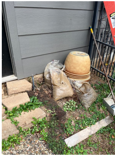
Example Rear Exterior Wall
