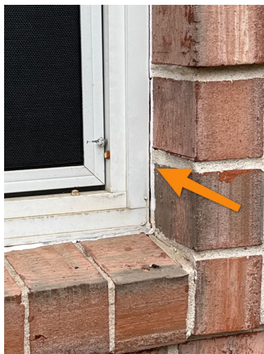
Example Right Exterior Wall
