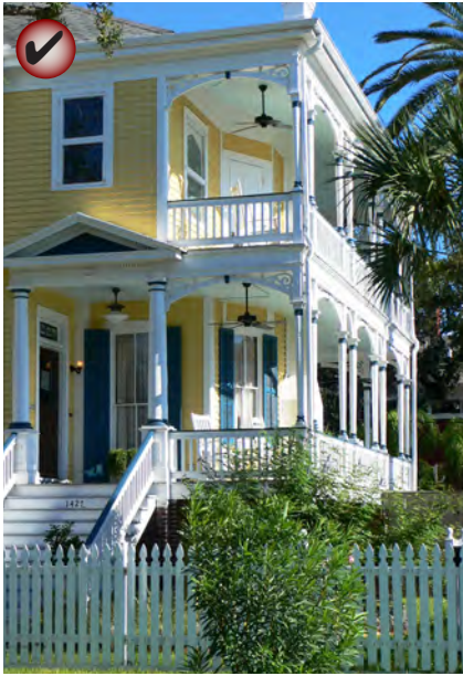
Maintain an original porch or gallery on a house.
