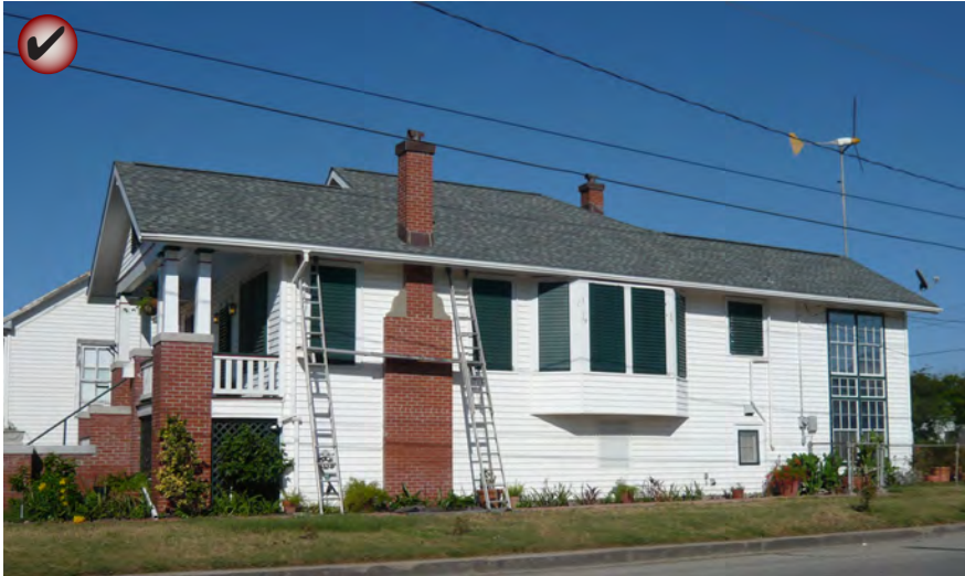
This house uses operable shutters, a sun room and wind generator for energy efficiency.
