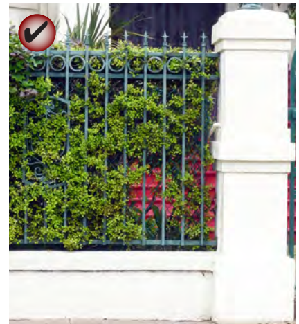
Maintain historically significant cast iron fences and stuccoed brick or concrete masonry site walls.
