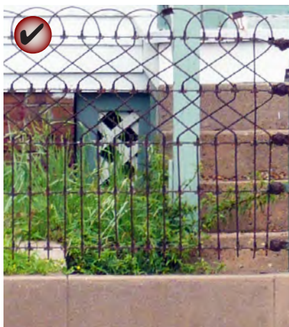
A simple wire fence is appropriate for use with some historic architectural styles.
