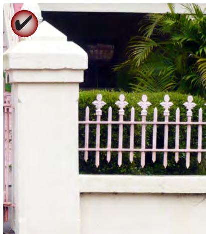
Maintain historically significant cast iron fences and stuccoed brick or concrete masonry site walls.
