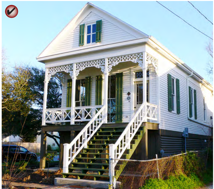
Where space allows, it is appropriate to extend front-facing porch stairs directly towards the street.
