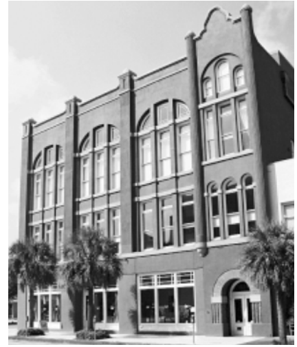
New construction in the Strand/Mechanic Historic District should maintain a strong, pedestrian-oriented street wall.
