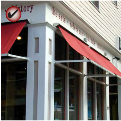
Install awnings to fit the window or door opening
