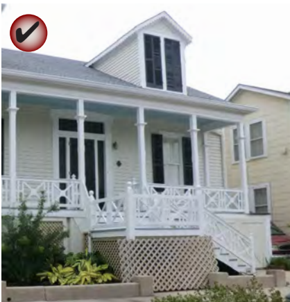
A 90 degree dog-leg stair extension may be appropriate to access an elevated front porch.
