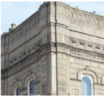
The façades of some historic commercial buildings in Galveston use stucco over brick to create the appearance of stone.
