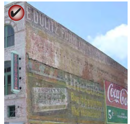
Historic painted wall signs, or “ghost signs” should be left exposed whenever possible.
