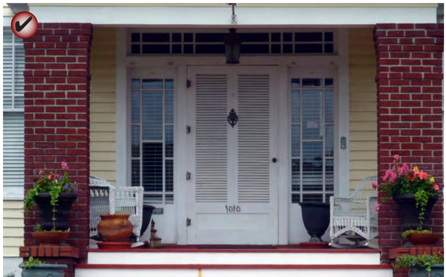
Use painted wooden screen and storm doors and louvered wooden doors that are backed with screening.
