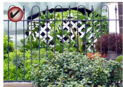
Metal loop and spear style fences are seen on a number of Galveston’s historic properties.
