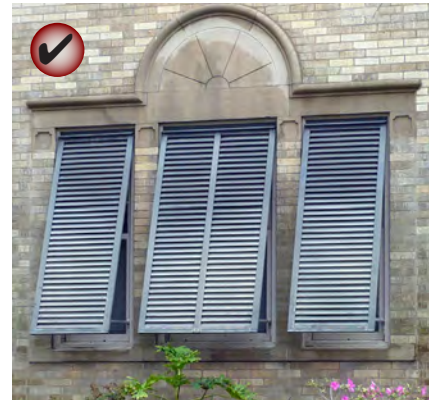
Preserve and repair existing wood shutters.
