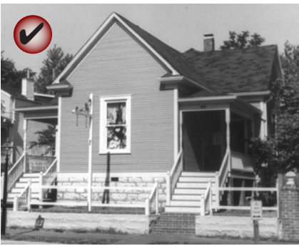
After: Original siding is revealed.
