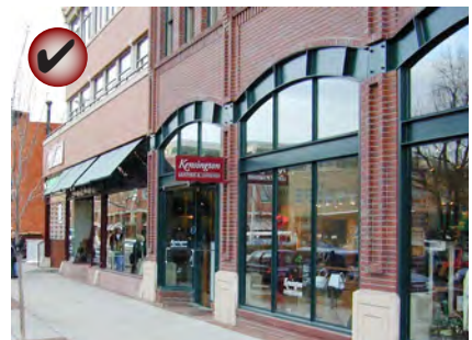
A new commercial structure in a locally-designated historic district should maintain the traditional pattern of recessed, front-facing entries.
