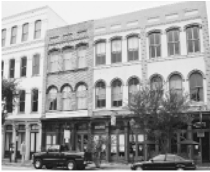
Commercial ground level storefronts align in a continuous horizontal bank; upper story windows create the same horizontal continuity.
