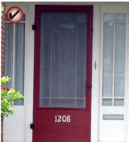
Use painted wooden screen and storm doors and louvered wooden doors that are backed with screening.
