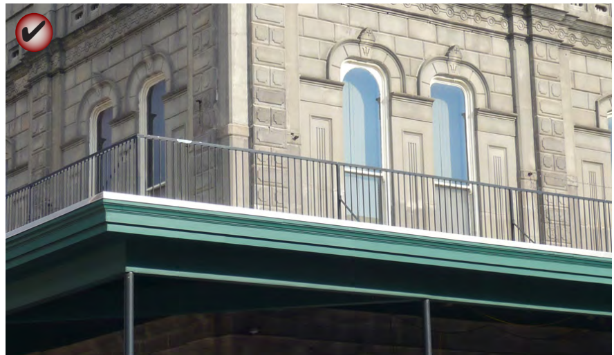
Design a new railing to be as transparent as possible so that it does not obscure the character-defining features of the building.
