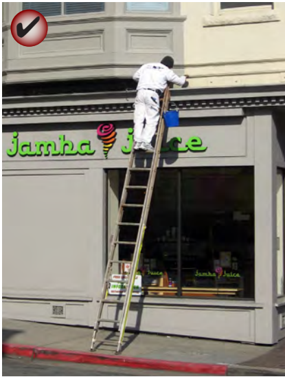
Repair deteriorated building materials.
