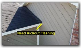
Observed a dead valley on the right side of the roof. There is no flashing installed to divert water away from the valley. Recommend a contractor evaluate and repair as needed.
