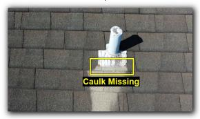
Observed damaged shingles in one or more areas of the roof. Recommend further evaluation by a professional roofing contractor.
