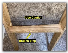
Observed damage to the attic access pull down.
