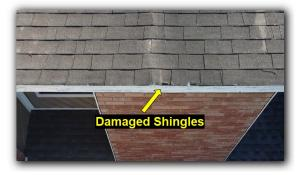
Observed excessive granule loss on multiple areas of the roof surface. Recommend further evaluation by a professional roofing contractor.
