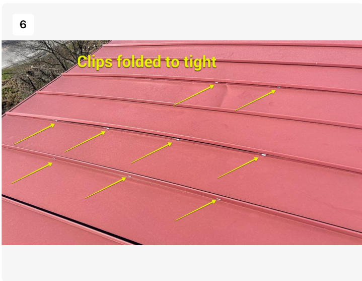
Clips are folded to tight and seam battens are disengaging.
