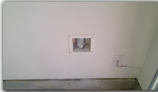
Location of main water supply valve: Inside the garage
