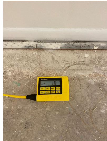
Right middle side of the slab
