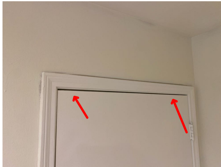
Front right bedroom door reveal
