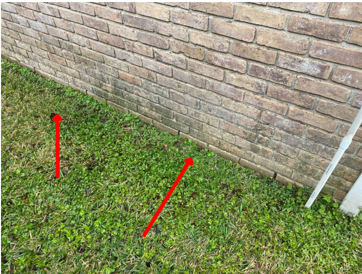
High Soil, Insuffieiant clearance to siding
