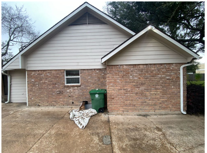
Left side of the house
