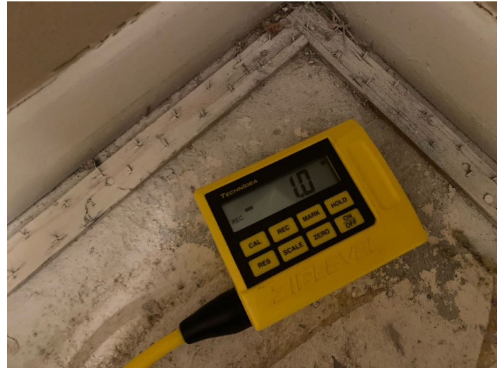
Front middle of the slab
