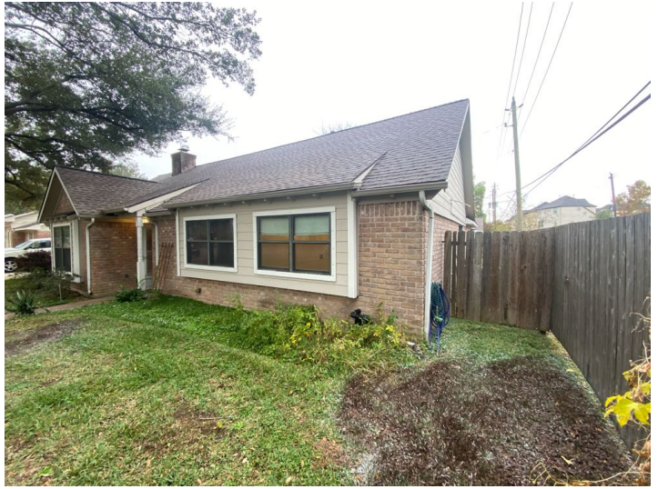
Front right side of the house
