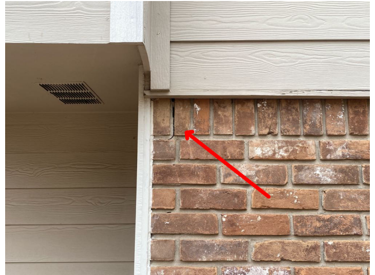
Mortar Crack
