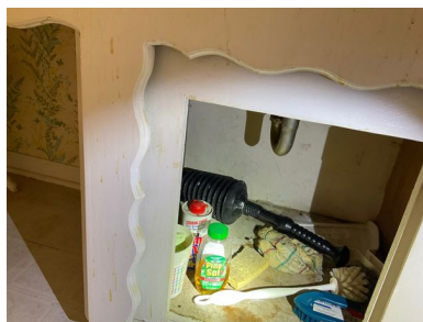
2nd Floor Bathroom
