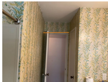
2nd Floor Bathroom
