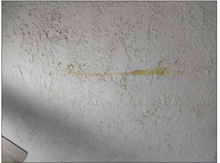
There are minor stains on the ceiling. Unable to determine condition of the underlying materials. Mainly at - front left bedroom
