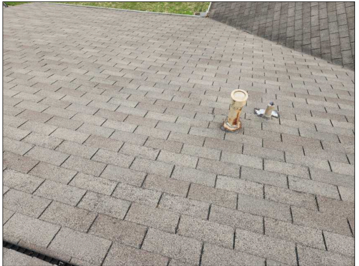
Overview of Roof.
