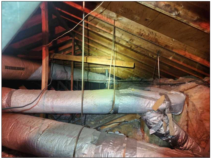
Overview of Attic.
