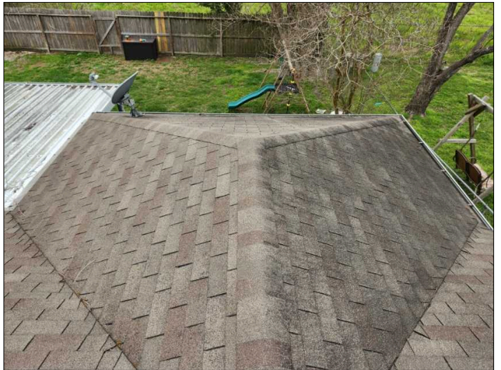
Overview of Roof.
