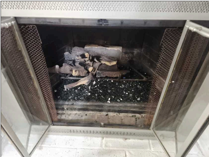
Overview of fireplace
