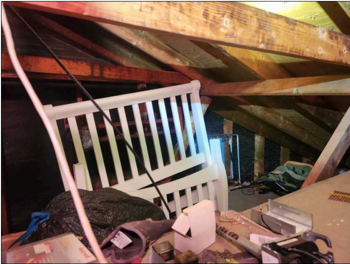
Overview of Attic.
