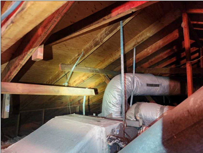
Overview of Attic.
