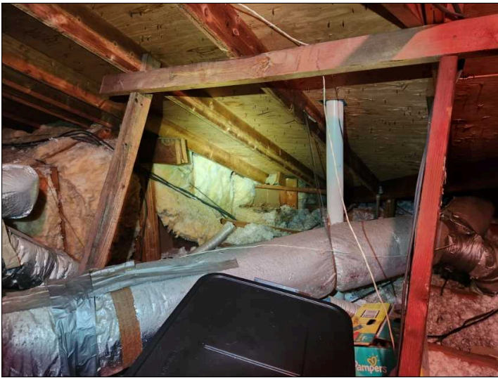
Overview of Attic.
