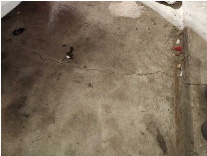
Cracks were noted in the pavement. These are cosmetic in nature at this time. Recommend sealing to help prevent further deterioration. Mainly at - garage
