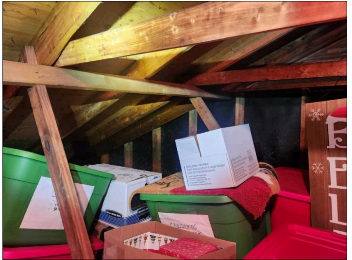
Overview of Attic.
