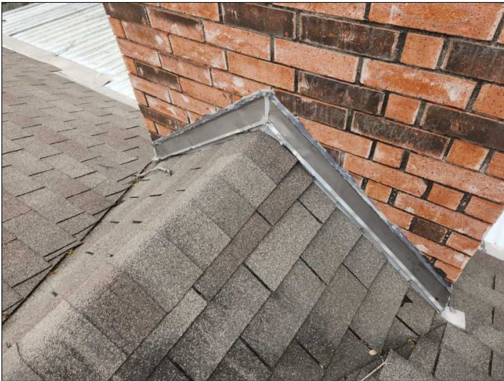
One or more of the vents and or flashing is unpainted, recommend painting all unpainted vents and flashing to help prevent damage due to UV rays or rust.
