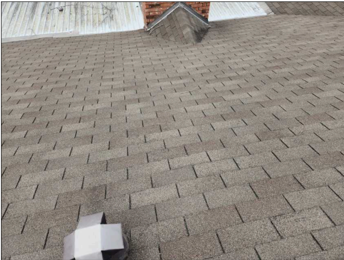
Overview of Roof.
