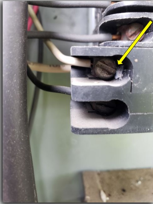
Abandoned wiring (national code says abandoned wiring should be removed from the panel).
