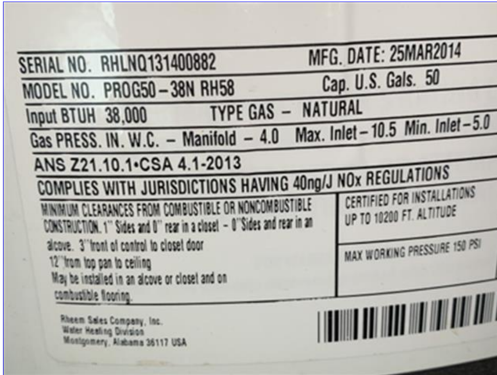
C. Photo 1(Picture) Water heater service tag.
