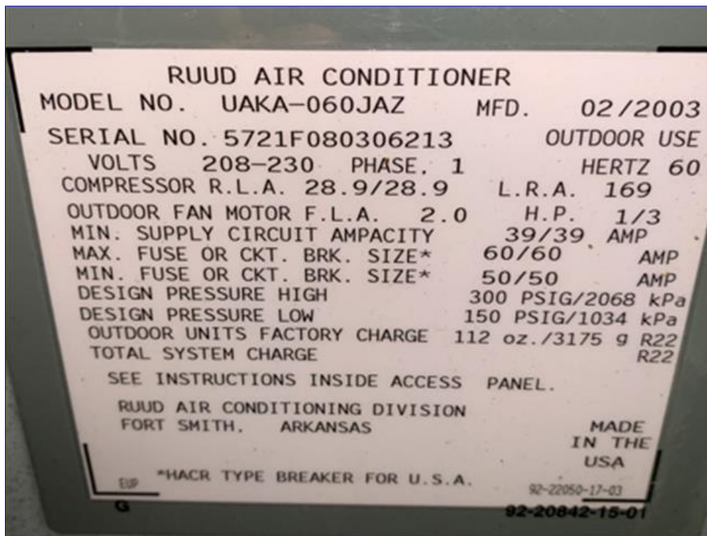
B. Photo 2(Picture) Air conditioner service tag.
