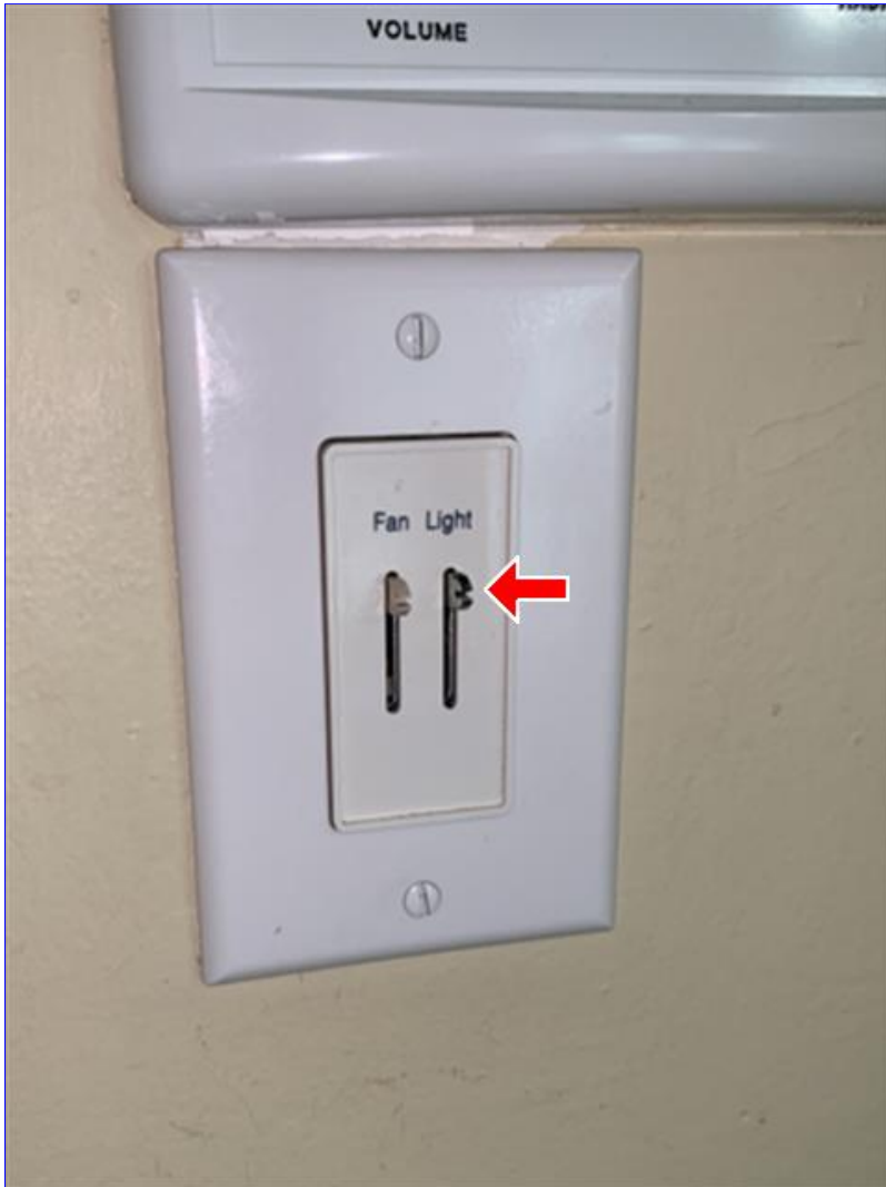
B. Photo 4(Picture) Several of the dual dimmer style light switches are missing the caps.
