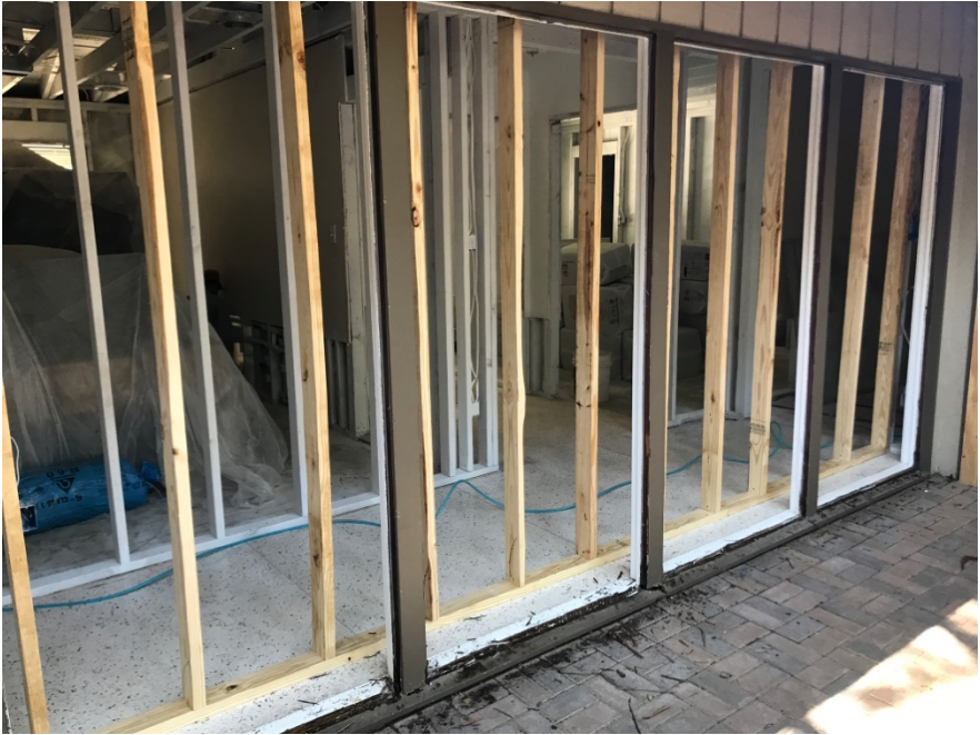
Windows in hall were removed and reframed.
