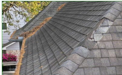
C. Item 3(Picture) Roof covering materials
