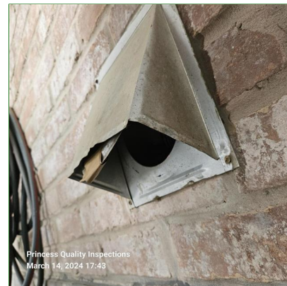
C. Item 2(Picture) The downdraft ventilation was performing at the time of inspection.
