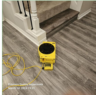
A. Item 2(Picture) Zip level spot check of foundation for level
