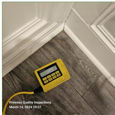
A. Item 16(Picture) Zip level spot check of foundation for level
