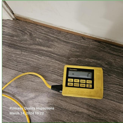
A. Item 5(Picture) Zip level spot check of foundation for level
