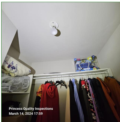
B. Item 2(Picture) Globes/covers are not present on light bulbs in closets.
