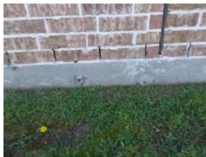
exposed cable end
