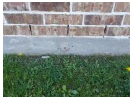
exposed cable end
