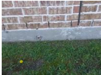
exposed cable ends rear
