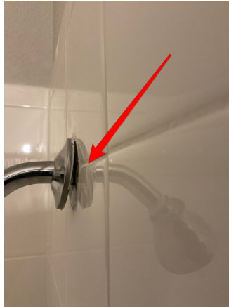
Public bathroom shower
