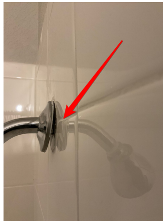
Public bathroom shower
