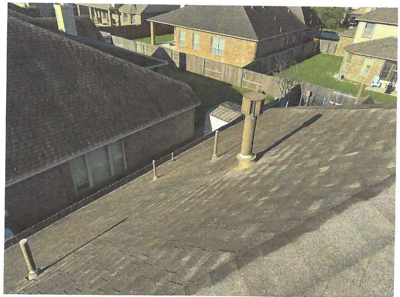
Photo Description: Vent flashings need paint
