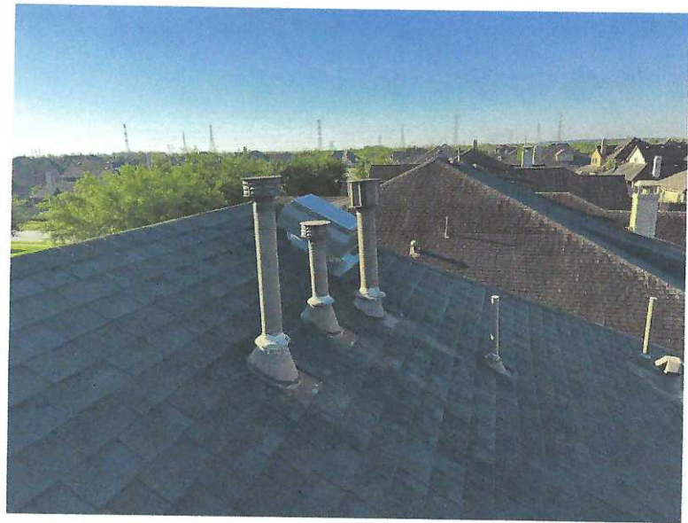
Photo Description: Vent flashings need paint
