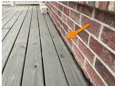
2nd Floor Deck
