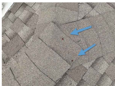
Garage Roof Level
