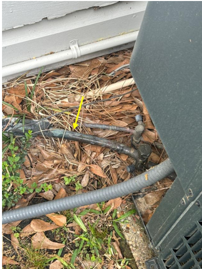
Insulation was deteriorated on the freon suction lines, in the attic/exterior.
