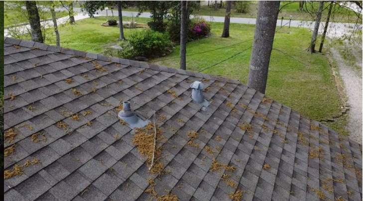
Structural Systems Roof Covering Materials
