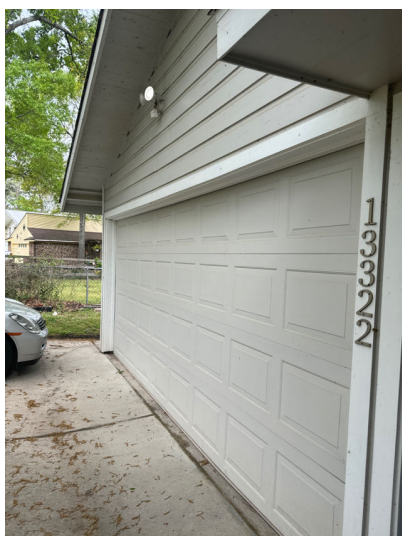
Structural Systems Walls (Interior and Exterior)
