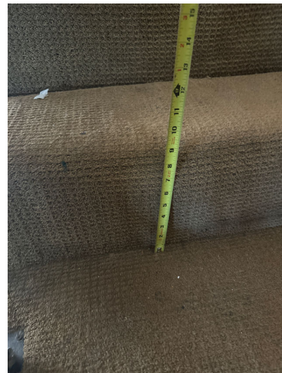
Stair landing was not 36 x 36 inches on each side. Stair risers were taller than the standard 7.5 inch height.
