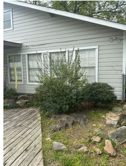
Structural Systems Walls (Interior and Exterior)
