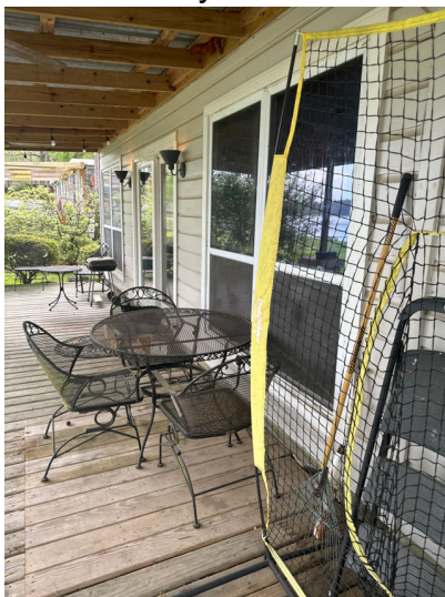
Structural Systems Walls (Interior and Exterior)
