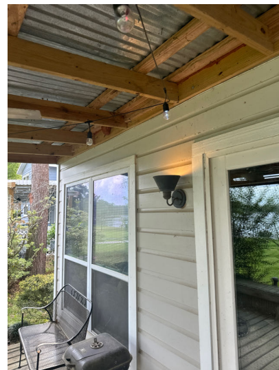
Structural Systems Walls (Interior and Exterior)
