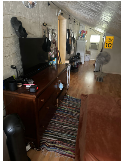
The limited height of the ceiling decreases the usable living space in the upper left bedroom.
