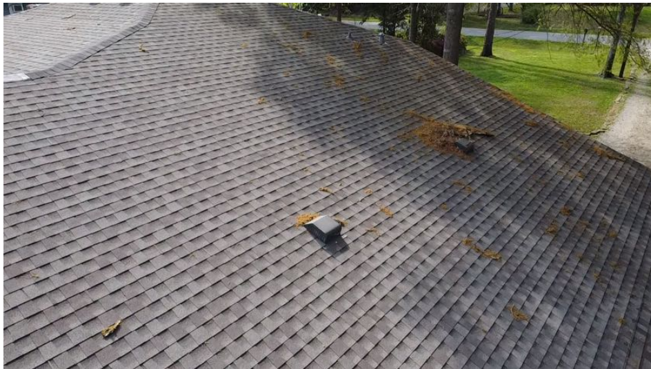
Structural Systems Roof Covering Materials
