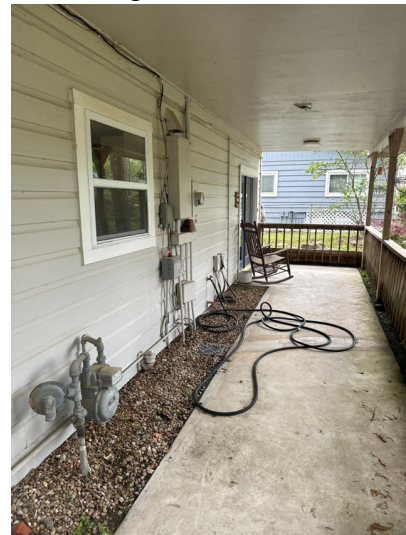
Structural Systems Walls (Interior and Exterior)
