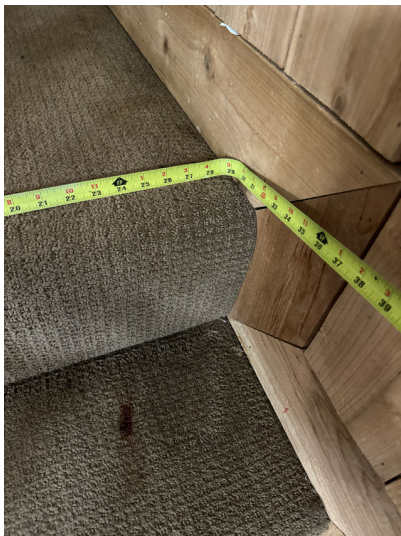
Stair landing was not 36 x 36 inches on each side. Stair risers were taller than the standard 7.5 inch height.
