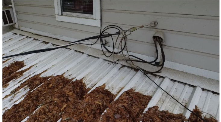
Drip loops on the service entry cable should be kept from touching the metal roof.
