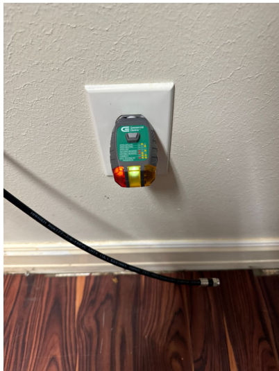
Outlet wiring in the lower bedroom was not correct.
