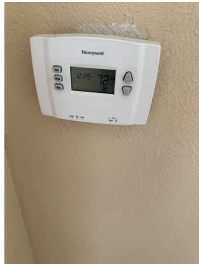
Thermostats were Honeywell type digital programmable located in the upper and lower levels.
