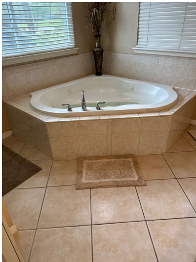
It did not appear that the hydro-massage equipment was GFCI protected.
