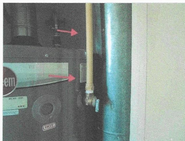
drip leg not gravity fed
