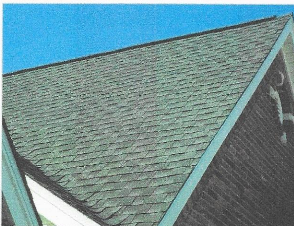
view of roof
