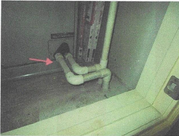
missing insulation
