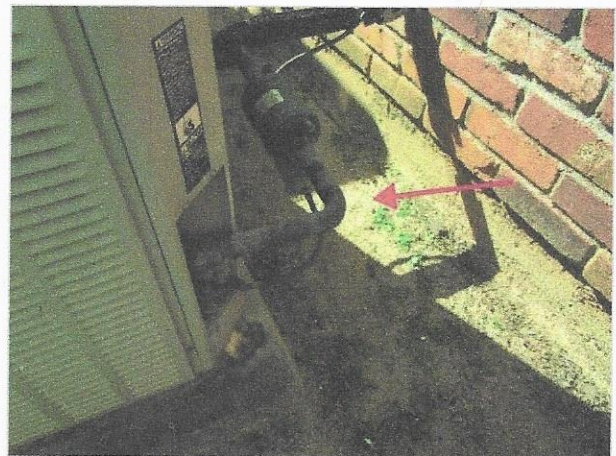
missing insulation
