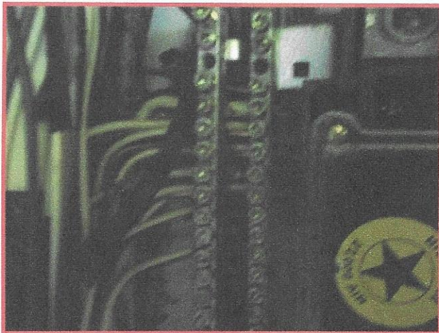
Double Tapped Neutrals on Buss Bar
