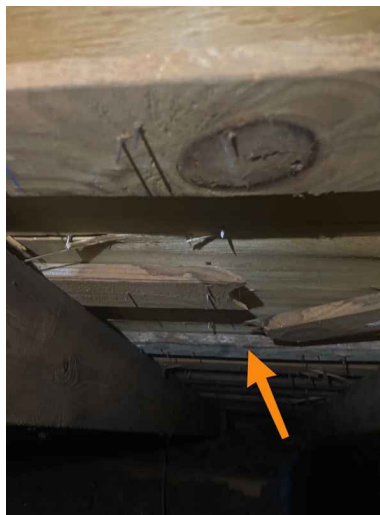
2nd Floor Bedroom Attic
