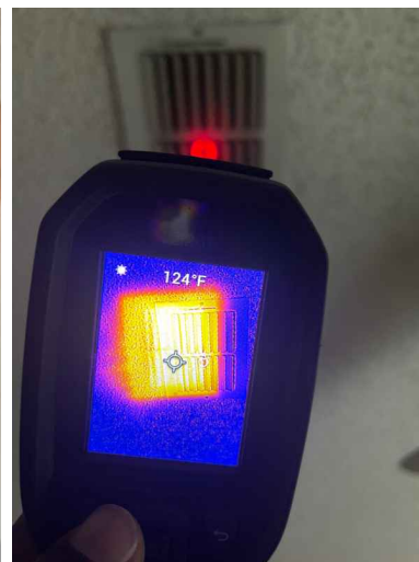
2nd Floor Rear Left Corner Bedroom
