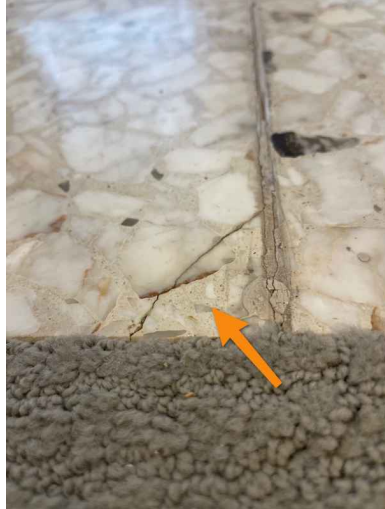
2nd Floor Jack & Jill Bathroom
