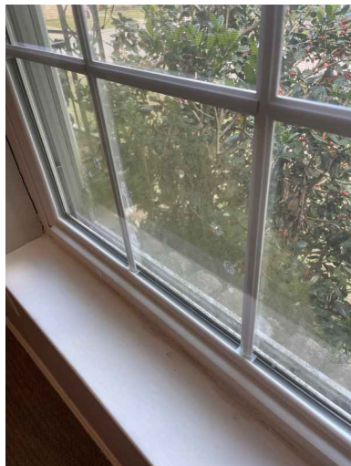
2nd Floor Front Left Corner Bedroom
