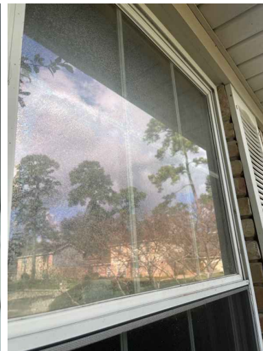
1st Floor Front Right Corner
