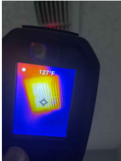
2nd Floor Front Left Corner Bedroom
