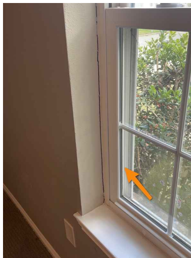
2nd Floor Front Left Corner Bedroom
