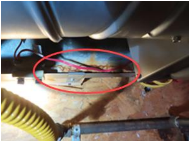
Little rust was observed in the evaporator coil overflow pan
