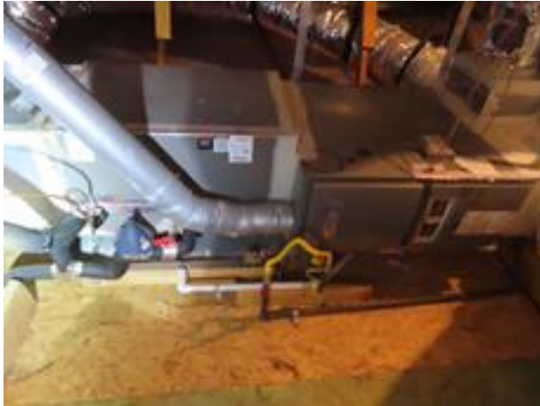
Info: Two LENNOX furnaces locate in the attic
