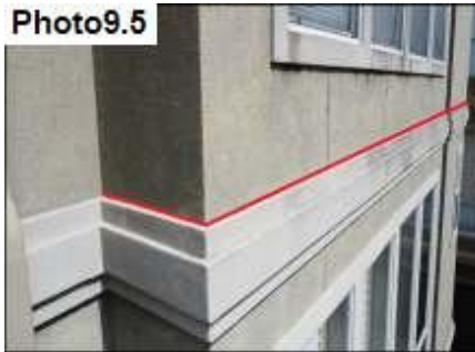
Foam Accent & Stucco Termination / Seal
