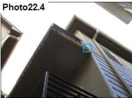
Balcony Flashing / Seal
