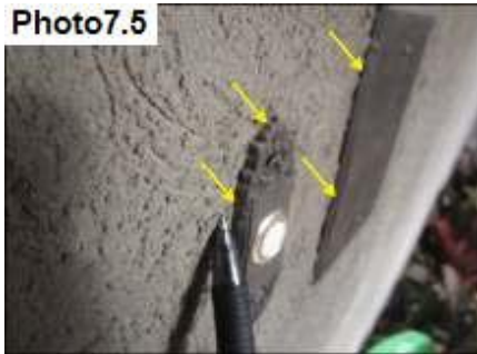
Penetration Sealants / Seal
