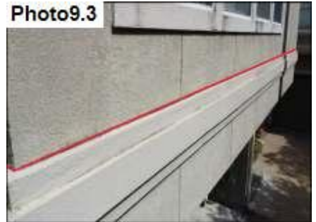
Foam Accent & Stucco Termination / Seal
