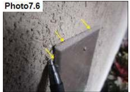
Penetration Sealants / Seal
