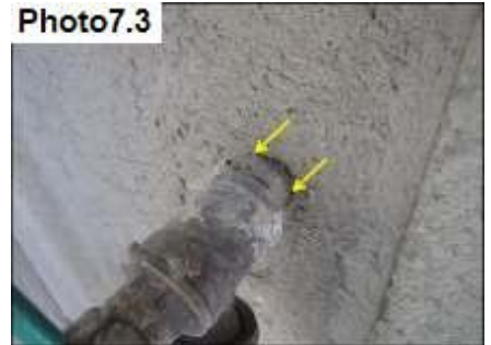
Penetration Sealants / Seal
