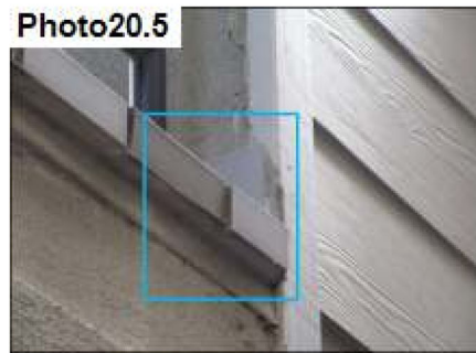
Balcony Flashing / Seal
