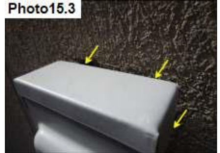
Penetration Sealants / Seal
