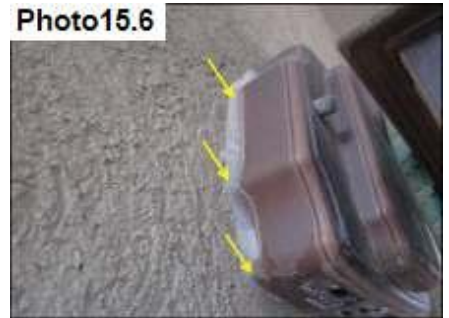
Penetration Sealants / Seal
