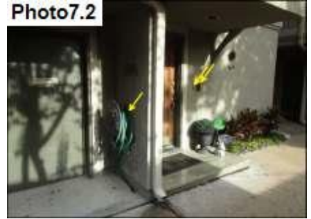
Penetration Sealants / Seal
