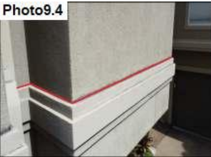
Foam Accent & Stucco Termination / Seal
