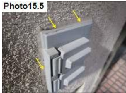
Penetration Sealants / Seal
