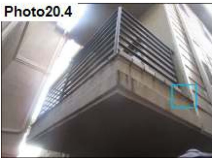
Balcony Flashing / Seal
