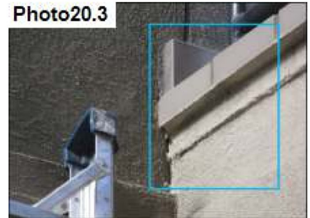
Balcony Flashing / Seal
