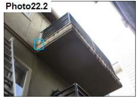
Balcony Flashing / Seal
