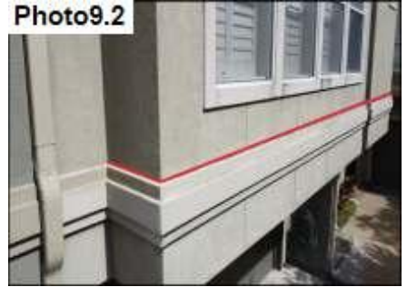
Foam Accent & Stucco Termination / Seal
