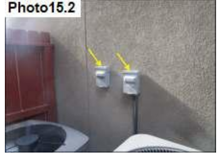
Penetration Sealants / Seal
