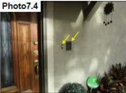
Penetration Sealants / Seal
