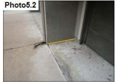
Stucco In Contact with Grade/ Apply a Kant Bead
