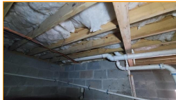
Main clean-out noted; The inspector is not required to open the main cleanout
