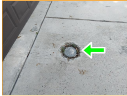
Main clean-out noted; The inspector is not required to open the main cleanout
