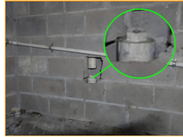
Sub-cleanout in the walls
