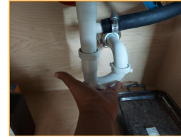
Inspecting under-sink plumbing in the primary bathroom
