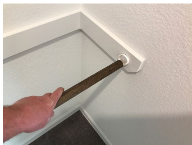
Rear Bathroom Closet
