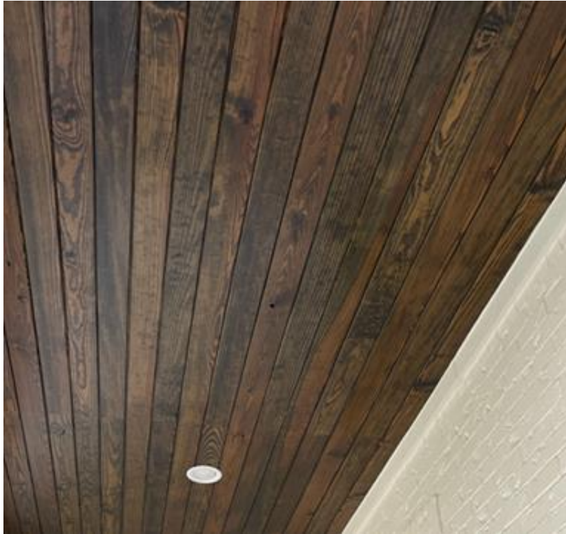
Front Porch & Back Patio Covering Ceilings: Wood Stained Mocha 280 (Oil Based) -- duplicated from the Sienna Model
