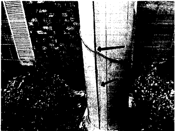
Damage to wood columns at front porch area at time of inspection
