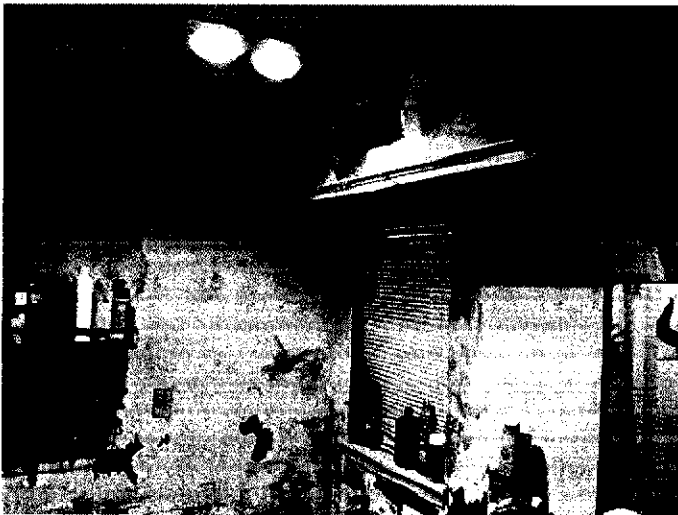
Light fixture above the toilet was nonoperational the time of inspection
