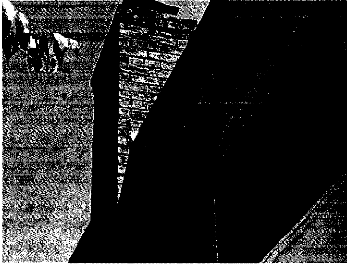
Soffit appears to be loose by chimney at left rear corner on second story at time of inspection
