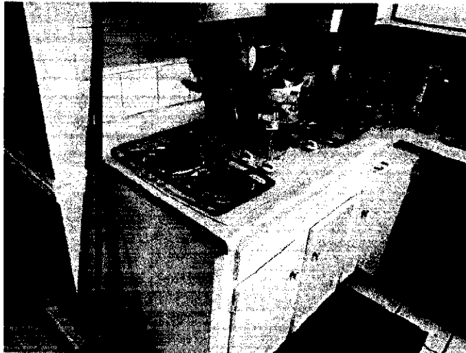
Cooktop was non-operational at time of inspection
