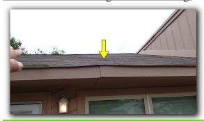
Lower side of flashing is not sealed down, wind driven rains can cause water penetration.
