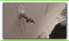
Exterior hose spigot(s) do not have code approved anti-back flow devices installed.
