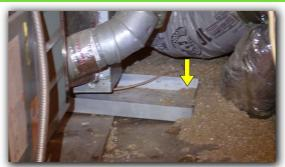
The air conditioner produces a differential temperature of 23.6 degrees F. Temperature differential is too great, indication of possible air flow restriction across coil and/or low Freon charge, needs service.
