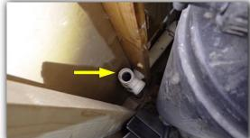
Escutcheon missing where plumbing penetrates the wall. Covering this penetration hole may help prevent air leaks and pest entry.
