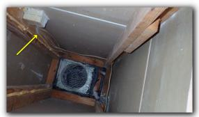
Observed possible micro-organism growth on air supply grills / vents which may be a concern due to increased awareness of environmental issues associated with molds. *If* this is a concern or potential concern, Texas House Check recommends contacting us for a mold testing, etc. Suggest replacing vents and registers.
