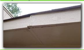
Need sealing / caulking around all holes and exterior siding penetrations on top and both sides, (*leave bottom open*) to prevent water entry. Including but not limited to dryer, bath and range top vents, light fixtures, etc.
