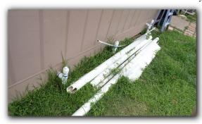
Some plumbing lines were rerouted due to relocating of the washer and dryer and installed in a manner to avoid removing cabinets and drywall.
