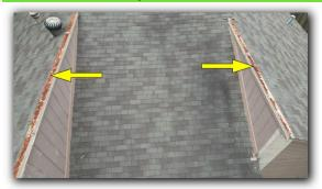
Sag(s) in roof decking observed. Probable cause is from improper/ inadequate framing in the attic or rotted/damaged roof sheathing.
