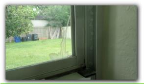
Front windows are very loose, appear to two separate windows improperly installed together.
