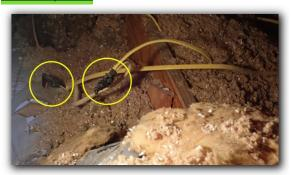
Multiple lights found to be not functioning. Probably just burned out bulbs, or it could be a broken fixture / switch or improper wiring. Observed at but not limited to the previous garage area.
