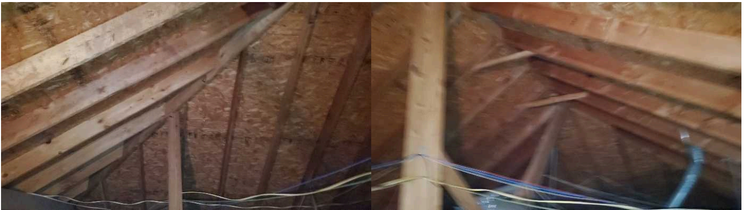
Picture of attic space
