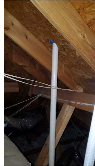
Drain line in the attic.
