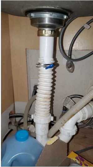
One or more of the sink have accordion-style flexible drain pipe installed (also sometimes called flexible waste pipe). These drains are known to trap solids in the ridges and split along the seams. Recommend replacing with PVC piping.
