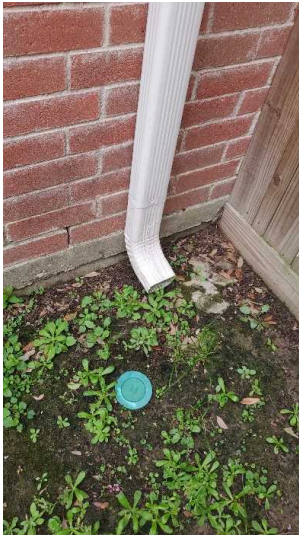
Gutter downspout discharging too close to the foundation.
