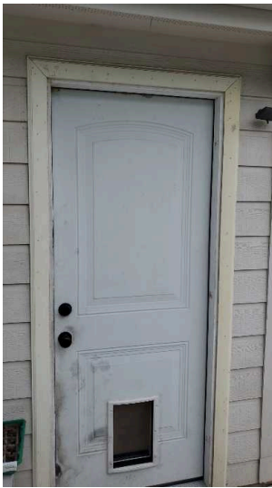
The exterior trim around the rear door is interior trim used on the exterior.
