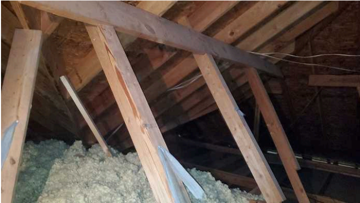
Picture of attic space
