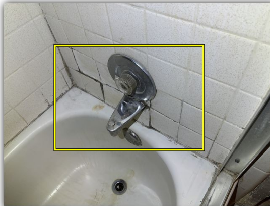
There is damage/cracking to the tub walls at the faucets. Water is leaking behind the shower wall and back wall of the hall closet.
