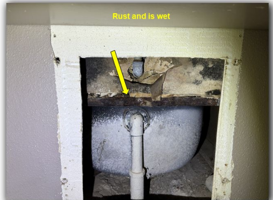
There is damage/cracking to the tub walls at the faucets. Water is leaking behind the shower wall and back wall of the hall closet.
