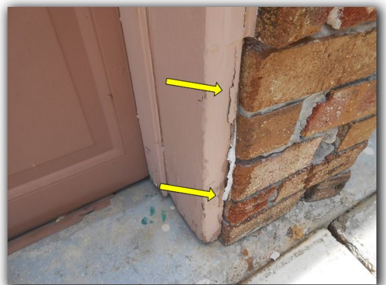
There are caulking gaps / deterioration at the trim around the garage door in more than one location.
