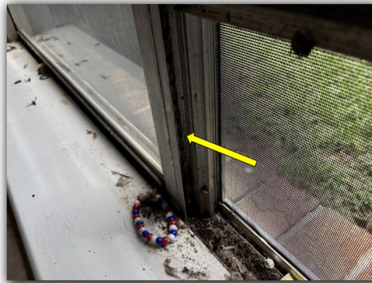
The springs have popped in the window frames inside the home at more than one location.
