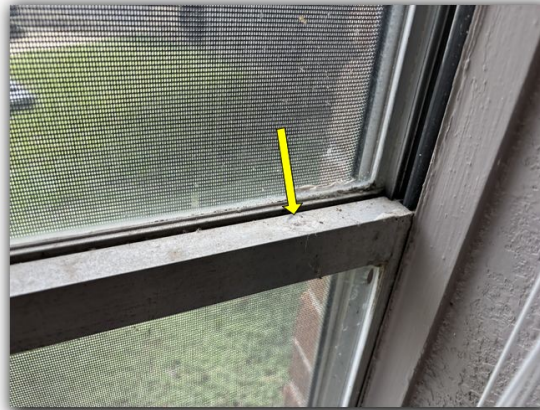
The springs have popped in the window frames inside the home at more than one location.
