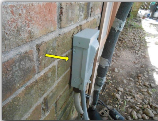
The A/C disconnect is not properly weather sealed on the exterior wall.
