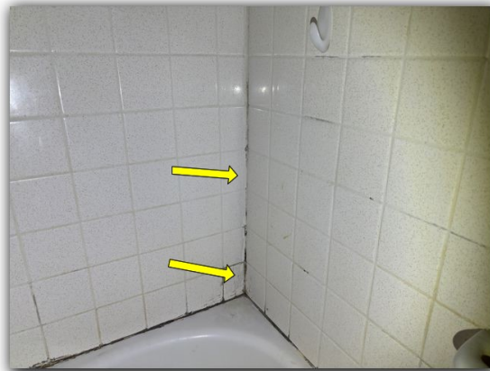
There is damage/cracking to the tub walls at the faucets. Water is leaking behind the shower wall and back wall of the hall closet.
