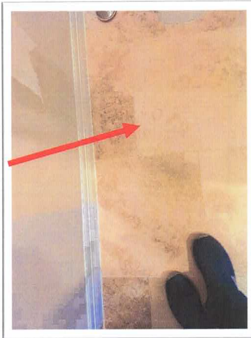
Cracks at cermaics in side of the main building
