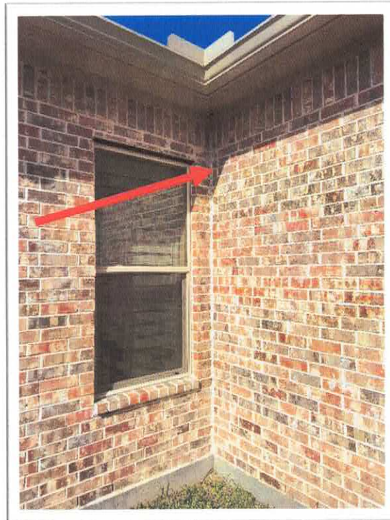
Crack at exterior wall corner
