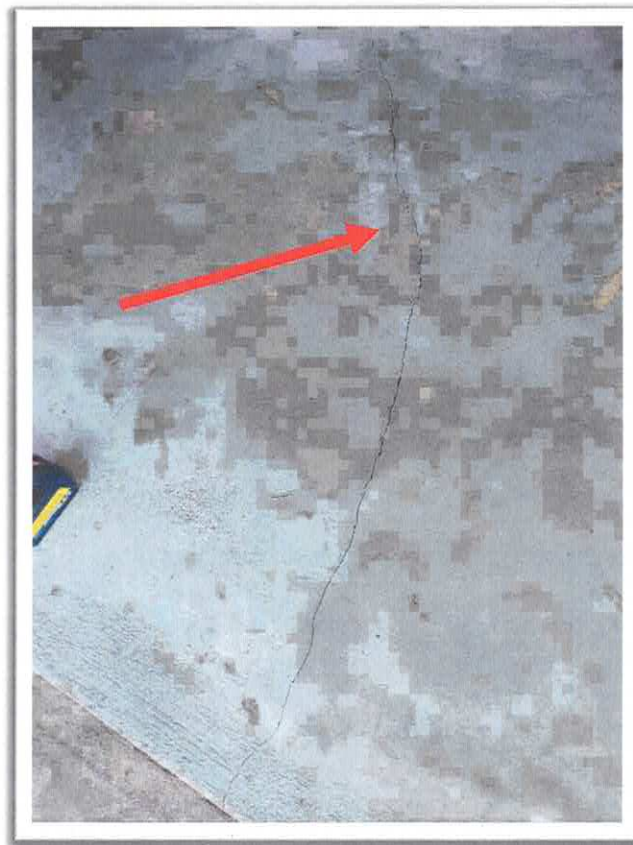
Foundation concrete crack at garage
