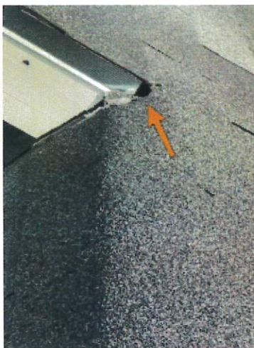
Breezeway to Garage
