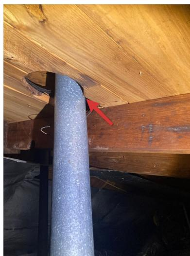
**2: Pan is missing or does not cover all possible leak area**
