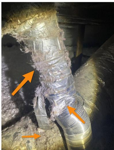
Venting material for dryer is damaged and exhausting lint into attic
