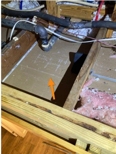
Insulation missing next to attic entry in master closet
