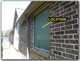
Note: It is sometimes difficult to determine if a seal is broken. For an exact number of broken seals, I recommend consulting a window professional.
