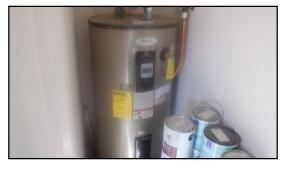
**At/near end of typical serviceable life.** Buyers note: The water heater(s) were observed to be over 10 years of age, multiple plumbing companies will only replace and are not likely to repair water heaters over 10 years of age.
