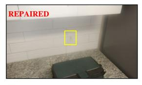
Did not observe GFCI protection of all outlets in required locations, including but not limited to the locations marked below. This condition is a recognized safety hazard and needs repair.
