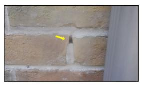
Caulking missing and/or deficient around windows / doors / vertical trim / joints in siding. May allow wind driven rain entry.
