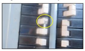
Not all breakers are properly identified. Per NEC E3606.2
