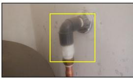
Drain line improperly reduced in size using a flexible connector, considered a recognized safety hazard; REF.: 1991 Standard Plumbing Code 1213.7.4 IRC 2803.6.1.
