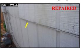
Observed one or more areas of damaged / cracked / chipped cement board siding.
