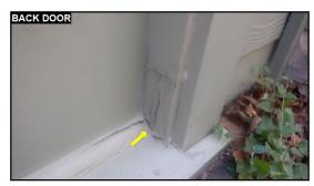
Improper threshold used on exterior doors without roof overhang protection from winddriven rains can result in water damage from intermittent water entry.
