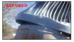
Damper missing required bracket that keeps damper from fully closing when the fireplace is equipped with gas logs. If the damper is fully closed then combustion fumes could enter house unseen.
