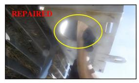
No electrical disconnect for electric water heater observed within sight. This does not comply with the current National Electric Code (NEC) minimum standards.
