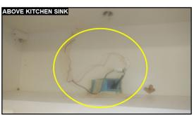
Electrical wiring run/routed too close to the attic access opening. This condition encourages damage to the wiring from personnel accessing the attic.
