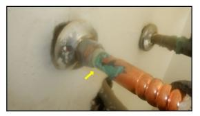
Located near house without benefit of a drain pan. Should water heater leak, interior finishes can be damaged.
