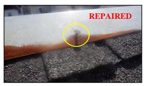
Observed spot repairs to the roof surface; possible water penetration area.
