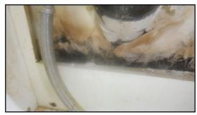
Water stains, damage or repairs observed, moisture meter indicated that stains are not active (wet) at the time of inspection; garage, powder bath.
