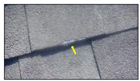
Standing water and/or stains from previous standing water observed on the flat roof. This condition is conducive to water penetration. Recommend roofer be consulted regarding the ability to correct drainage on the roof to prevent/reduce standing water.
