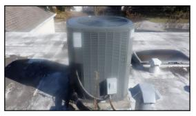
Electrical line supplying power to A/C outside is not fully enclosed in protective conduit.
