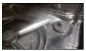
Drain line needs to be better elevated and secured above side inlet of disposal to prevent debris and gray water from draining down line from disposal and back into dishwasher.
