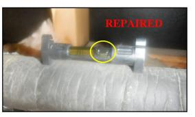
The primary drain line should be insulated along the entire length to prevent warm air condensing on the cool drain line and dripping condensation. Observed flexible drain line, these drain lines are easily routed up-hill and / or kinked / clogged. Recommend replacing with hard pipe.
