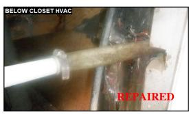
Could not verify primary drain line drains into a "wet" plumbing trap per today's industry standards. Could result in possible sewer gas and bacteria backing into HVAC equipment / ducts and into house.
