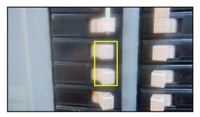
One or more breaker(s) were off at the time of inspection. Inspector does not turn on breakers found in off position due to potential short/electrical problem. Recommend inquiring seller regarding information regarding any/all breaker(s) found in off position.
