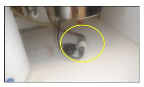
Improperly wired, 3 prong outlet not grounded or polarity reversed, including but not limited to; garage. powder bath.
