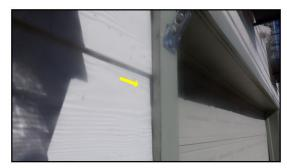
Need sealing/caulking around all holes and exterior siding penetrations on top and both sides, (*leave the bottom open*) to prevent water entry. Including but not limited to dryer, bath and range top vents, light fixtures, etc.
