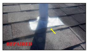
Observed rusted flashing at one or more locations. Recommend painting all exposed metal above roof line to prevent rusting and extend service life.
