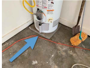
ELEVATION AND PHYSICAL PROTECTION OF WATER HEATERS INSTALLED IN GARAGES FIGURE 28-9
