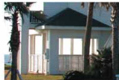
Louvered railing at ground level
