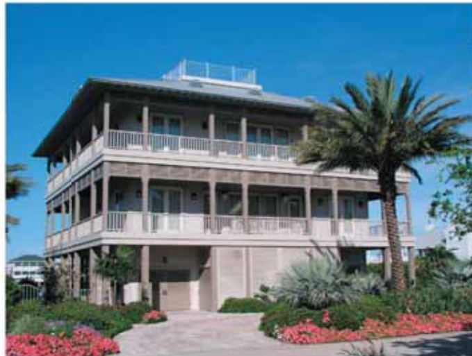
Elevated pile construction
