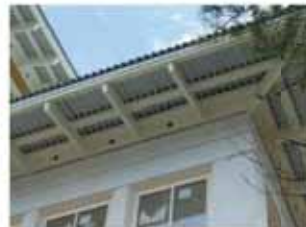
Exposed rafters, purlins and underside of deck
