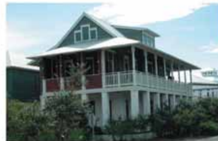
Traditional broken back roof
