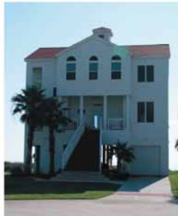
Overscaled entry stair
