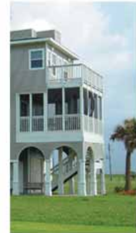
Porch integrated with structure
