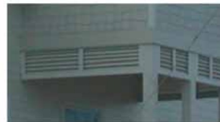
Apron between columns
