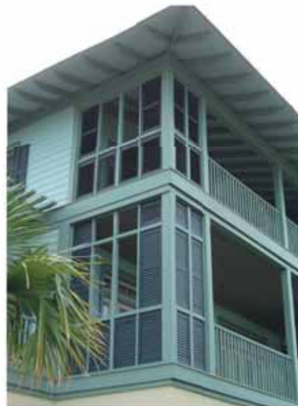
Painted porch, screens, railing and trim
