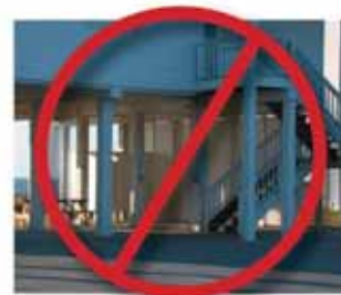
Uninhabitable ground level
