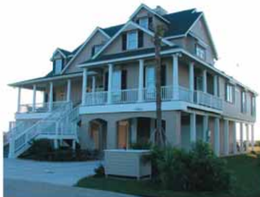
Elevated structure with wraparound porch
