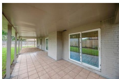
Closer View of Covered Patio
