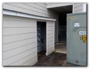
Sub Panel #1 Box Rating: 200 amps Box Location: Exterior Storage Room Cabinet Manufacturer: Power Master
