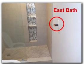
Two of the switches appear to be damaged and do not operate properly. The switch to the sconce light and the recessed lights in the living room did not operate.
