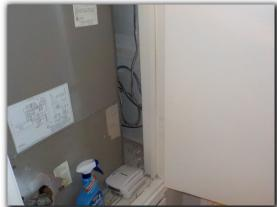
Not all of the bathroom receptacles appear to be connected to a ground fault circuit interrupter (GFCI) device. Under current electrical standards, all of the bathroom receptacles should have GFCI protection.
