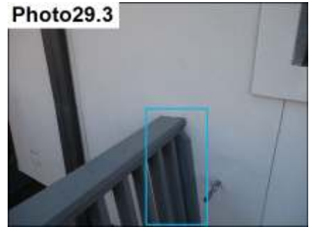
Railing & Stucco Termination / Seal
