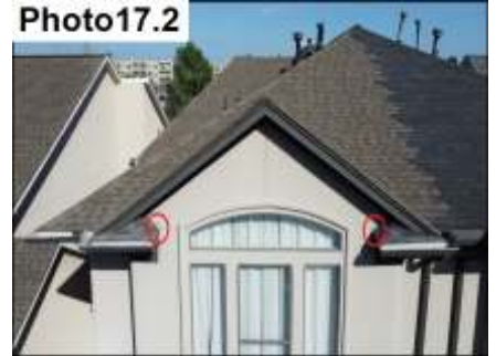
Roof Termination / Seal
