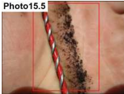
Substrate Damage / Assess, Repair & Install Relief
