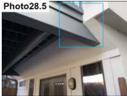
Balcony & Stucco Termination / Seal
