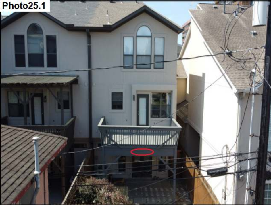
Missing Door Head Flashing / Install
