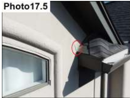
Roof Termination / Seal
