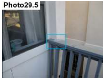
Railing & Stucco Termination / Seal
