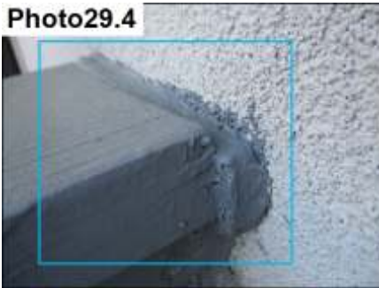
Railing & Stucco Termination / Seal
