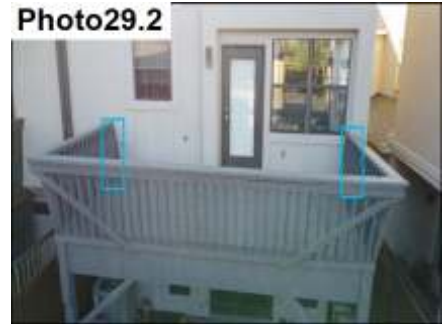
Railing & Stucco Termination / Seal
