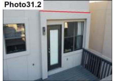
Flat Accent / Install Metal Cap or Apply Elastomeric Coating
