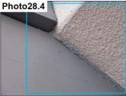
Balcony & Stucco Termination / Seal
