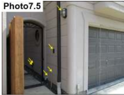
Penetration Sealants / Seal
