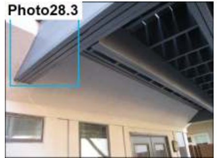
Balcony & Stucco Termination / Seal
