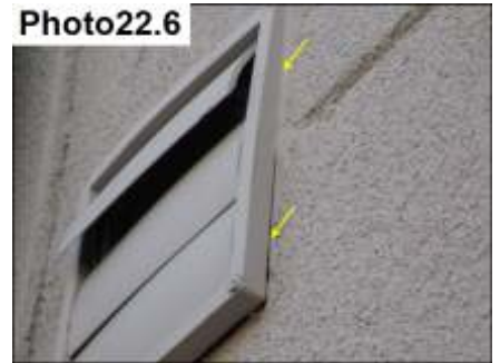
Penetration Sealants / Seal
