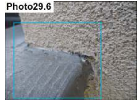
Railing & Stucco Termination / Seal
