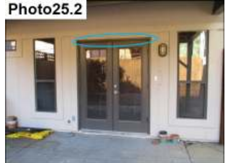
Missing Door Head Flashing / Install
