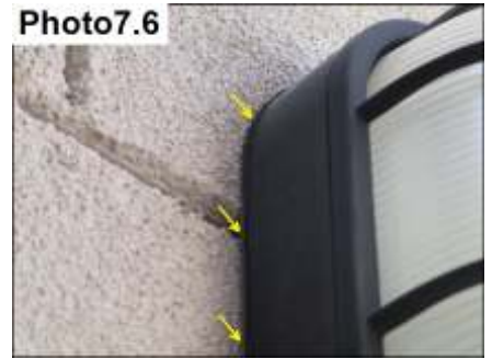
Penetration Sealants / Seal
