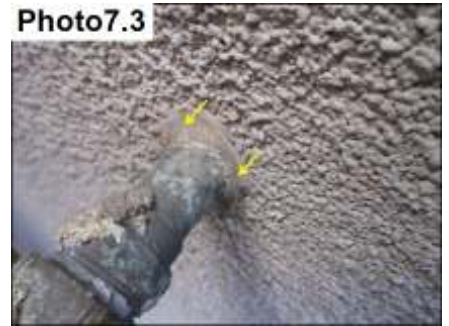
Penetration Sealants / Seal
