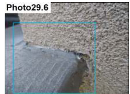
Railing & Stucco Termination / Seal
