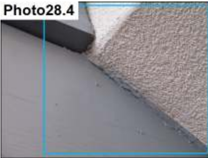
Balcony & Stucco Termination / Seal
