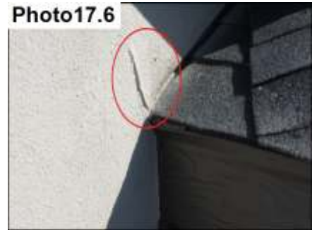
Roof Termination / Seal
