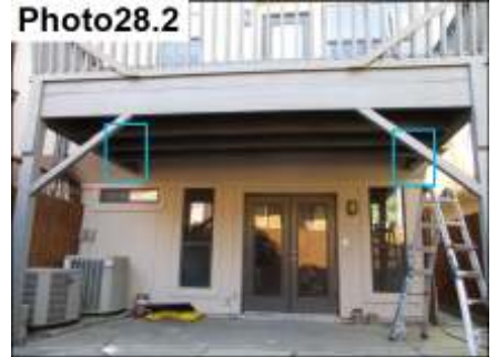
Balcony & Stucco Termination / Seal
