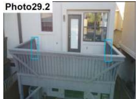
Railing & Stucco Termination / Seal
