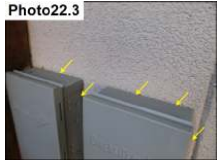
Penetration Sealants / Seal
