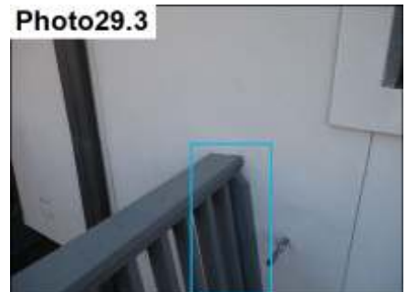
Railing & Stucco Termination / Seal
