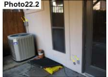
Penetration Sealants / Seal
