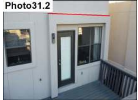
Flat Accent / Install Metal Cap or Apply Elastomeric Coating
