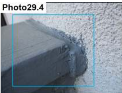
Railing & Stucco Termination / Seal
