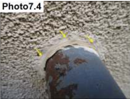
Penetration Sealants / Seal
