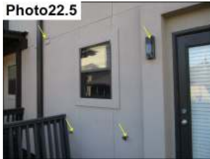
Penetration Sealants / Seal
