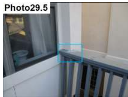
Railing & Stucco Termination / Seal
