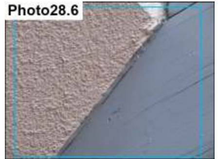
Balcony & Stucco Termination / Seal
