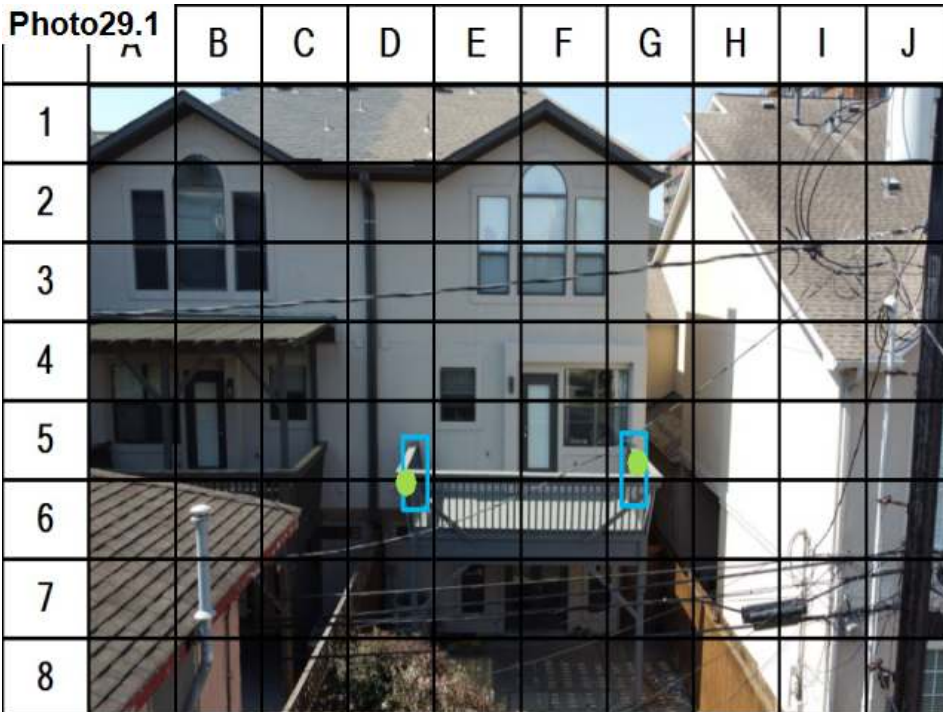
Railing & Stucco Termination / Seal
