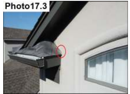
Roof Termination / Seal
