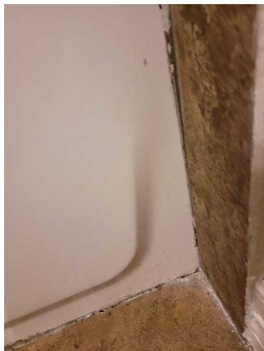
Primary Floor Front Hall Bathroom
