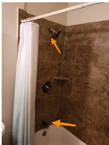
Primary Floor Front Hall Bathroom
