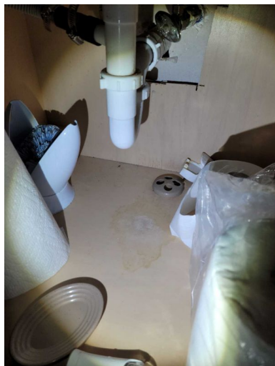
Primary Floor Hall Bathroom
