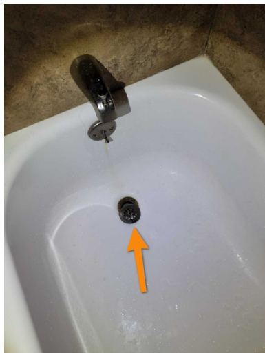
Primary Floor Front Hall Bathroom
