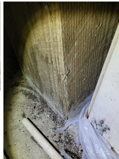
Garage Front Left
