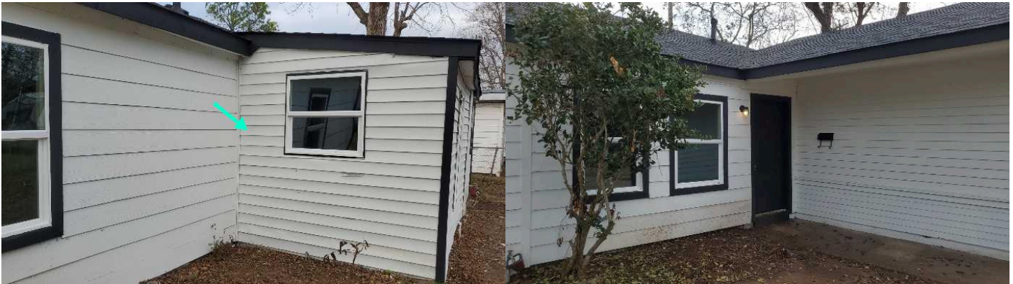
Vinyl siding on the rear addition.
