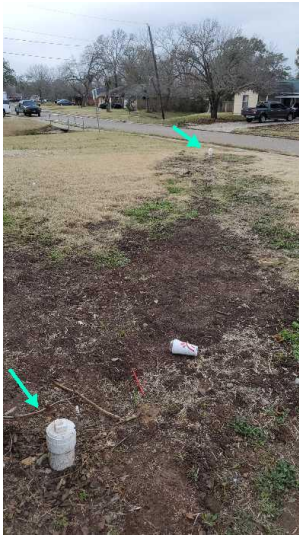
Drain line clean outs in the front yard.
