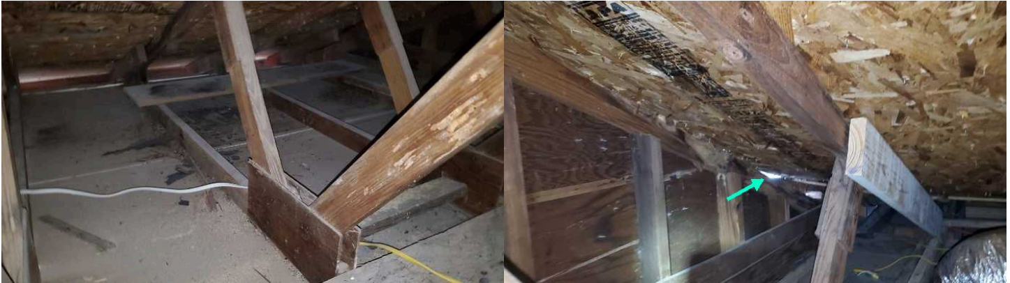
Missing insulation.
