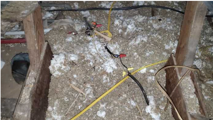
Multiple open wire splices in the attic. Wire splices should be contained in junction boxes to prevent contact with live wires.
