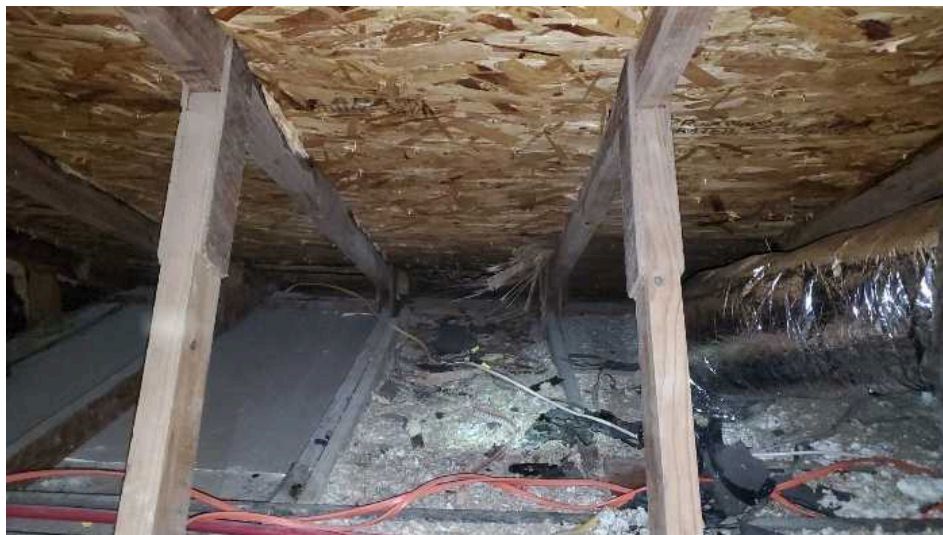
Multiple open wire splices in the attic. Wire splices should be contained in junction boxes to prevent contact with live wires.
