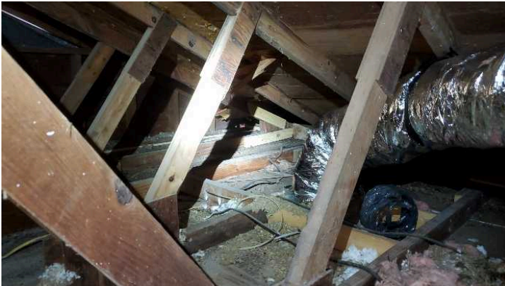
Missing insulation.
