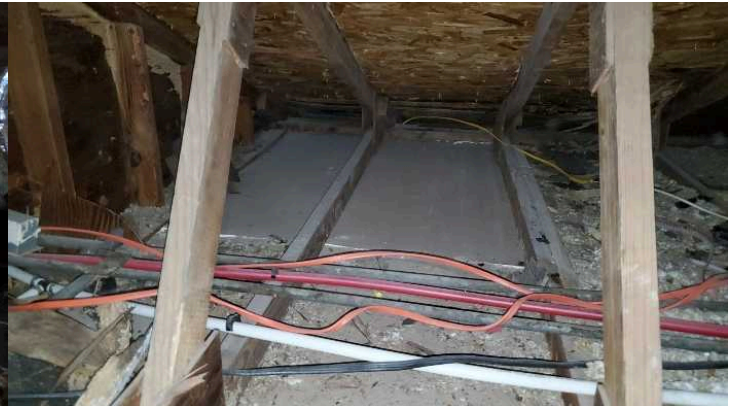
Missing insulation.
