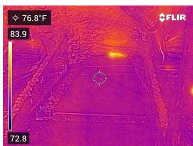
right side wall eaves
