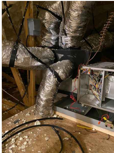
HVAC not Electrically Connected:
