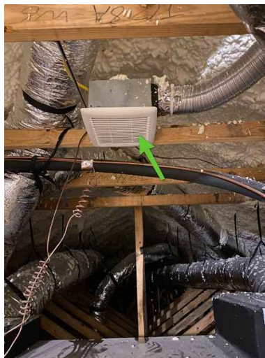
This is the continuously running attic ventilation fan to keep moisture down since this is a ventless, conditioned space. It exhausts along the right side wall under the eaves.
