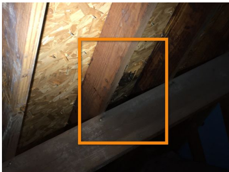
Southeast area of the attic
