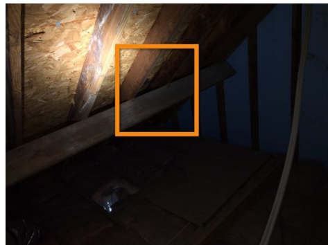
Southeast area of the attic
