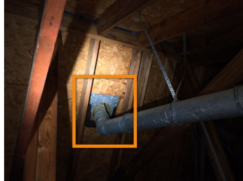
Furnace flue pipe at the west side of the attic
